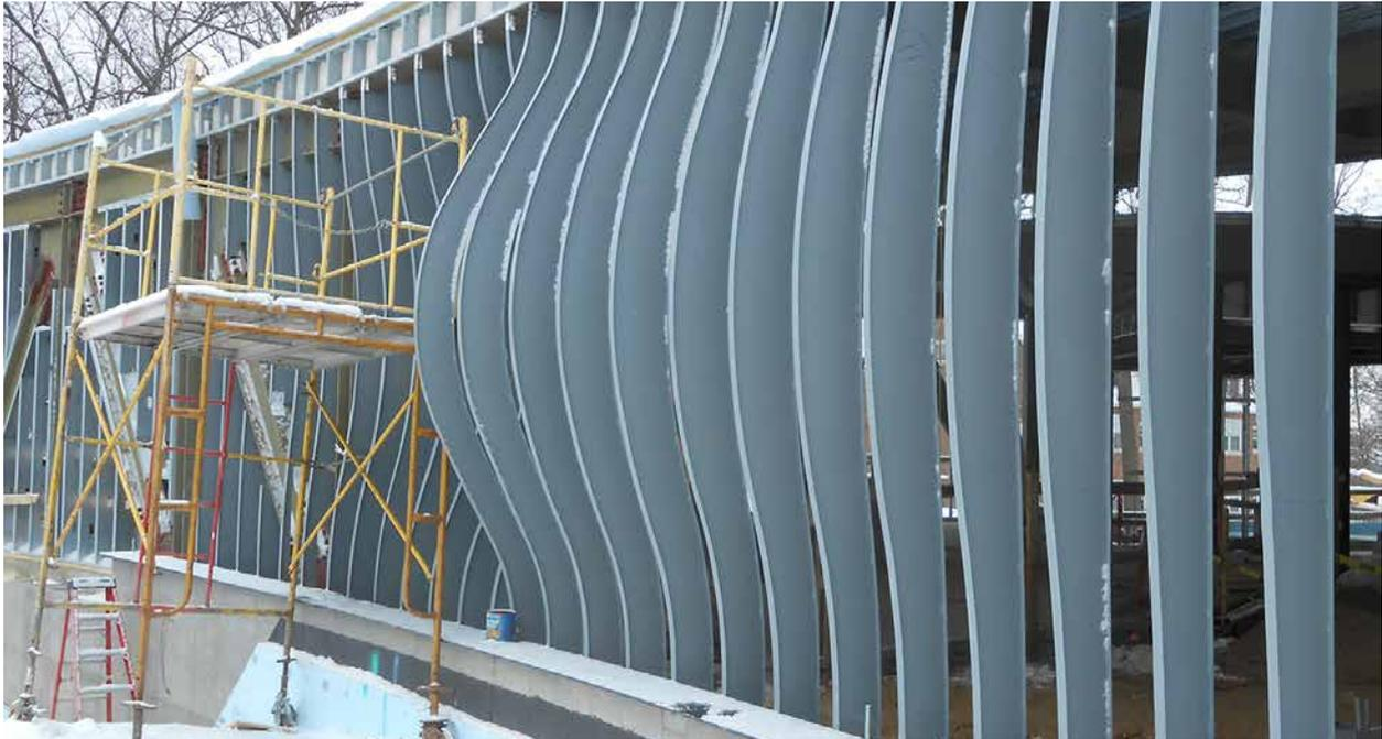
**16.12.** Specially fabricated metal studs shaped the “warped” wall. Credit: Studio Gang Architects.
