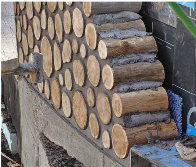
**16.8.** Typical exterior wood masonry walls are 11 inches thick, with a solid mortar joint. The other layers that make up the wall assembly are described in the text. Credit: Studio Gang Architects.
