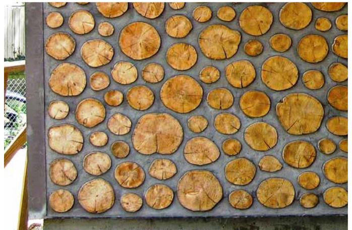
**16.14.** The masons maintained a good balance of log sizes throughout, while keeping a constant minimum width of mortar joint. Credit: Studio Gang Architects.
